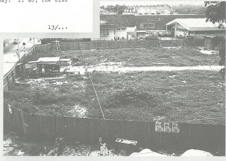
The Beginnings – Ground works in progress on the site (MMA House 1970)
